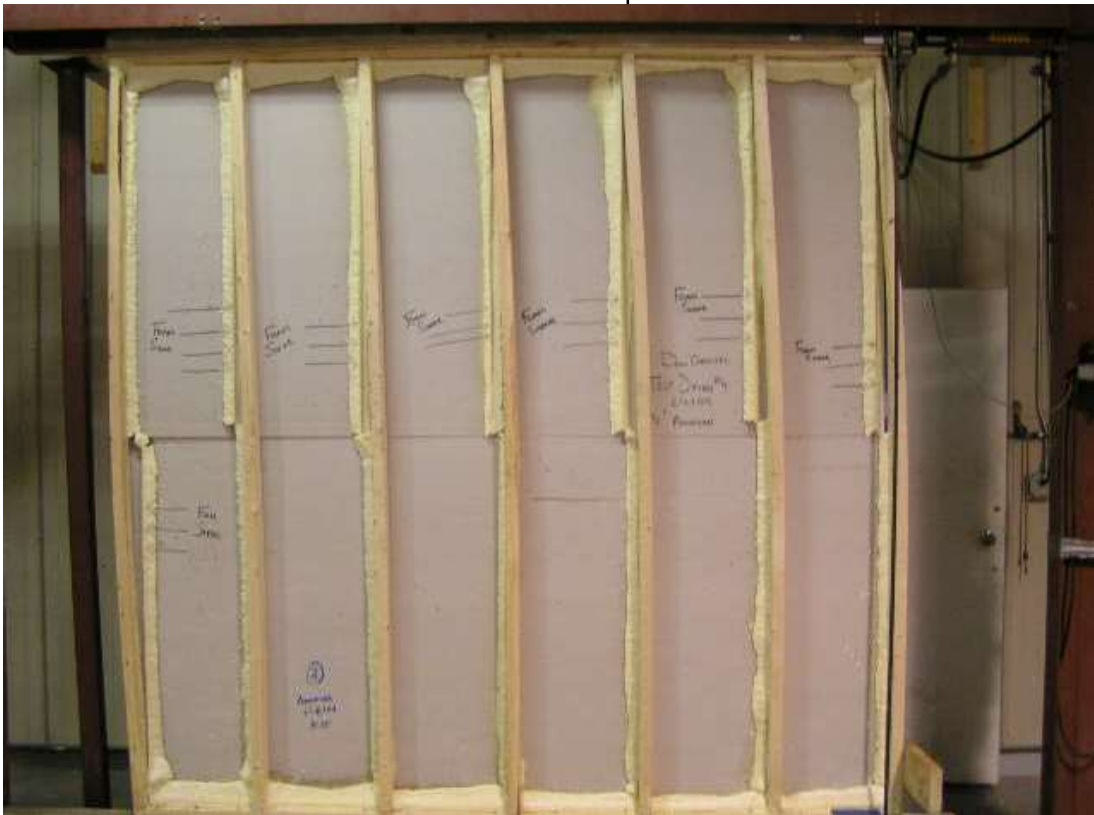
Test #1 Stud Failure
